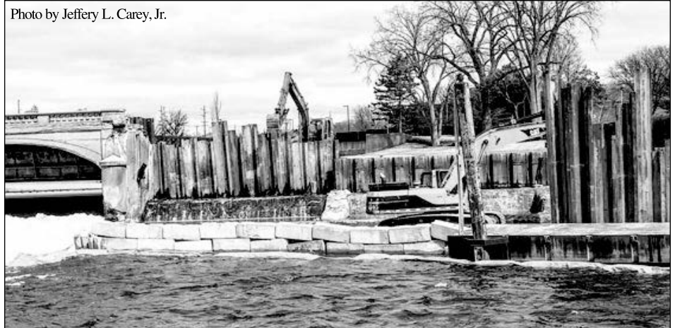
Backhoe removing rubble from demolished south quarter
