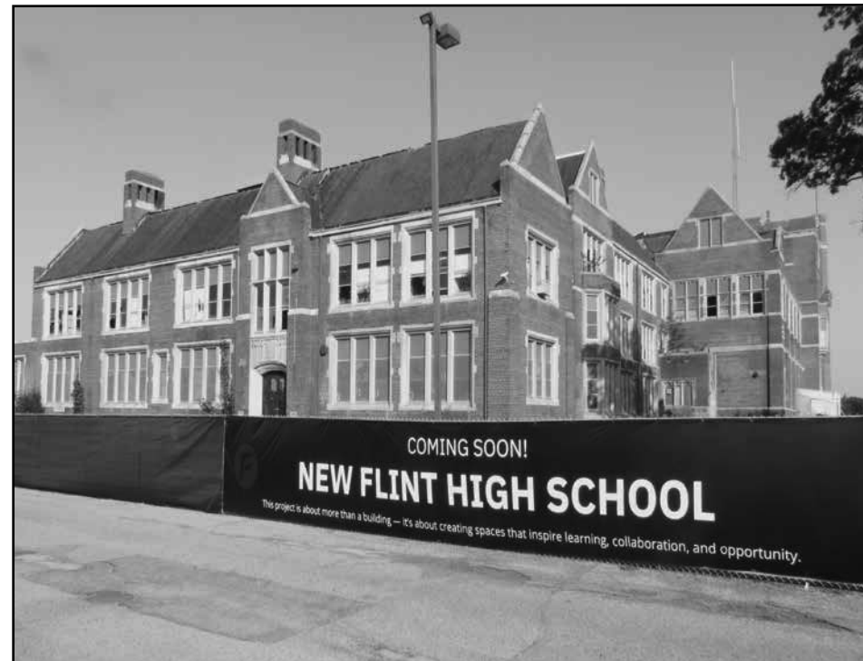
Abatement and demolition work have begun on the former Flint Central High School and Whittier Classical Academy structures. (Photo by Harold C. Ford)
